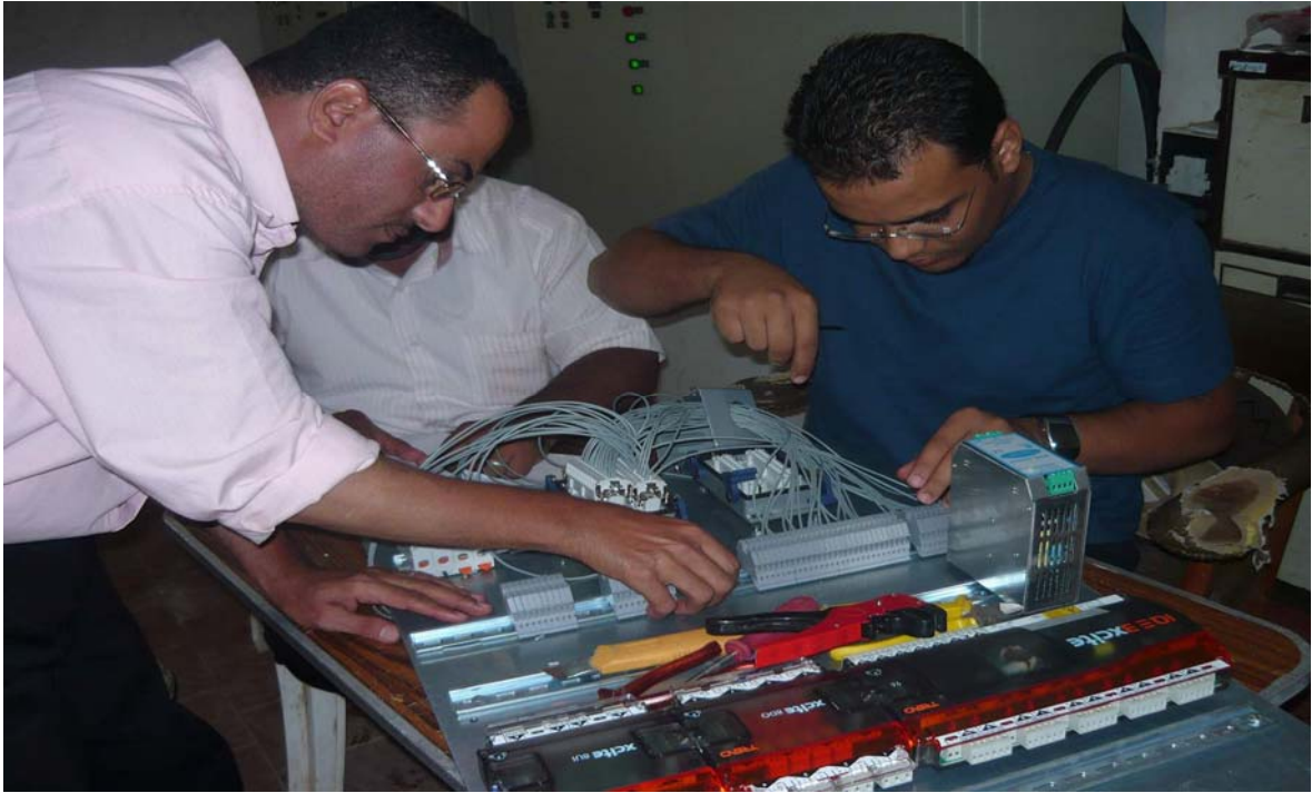
Control Panel Assembly
